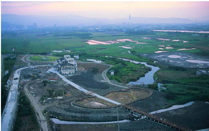
Source 7. Guandu Nature Park under construction (photo)
